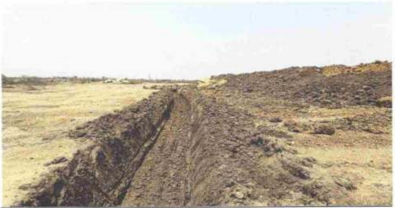
Catchment drain along the water harvesting pit
